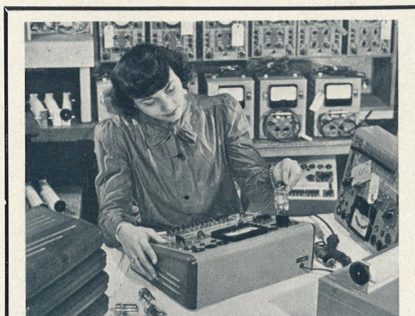
THIS PICTURE OF PATRICIA GREENE , inspector in Williamsport's Test Instrument Assembly Department, appeared in full color on the cover of last month's issue of Radio News. Pat is making a final check on one of Sylvania's latest products—its improved tube tester for radio servicemen.
